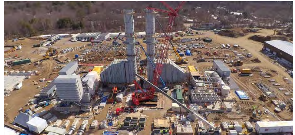
State-of-the-art peaking plant under construction at Medway.
