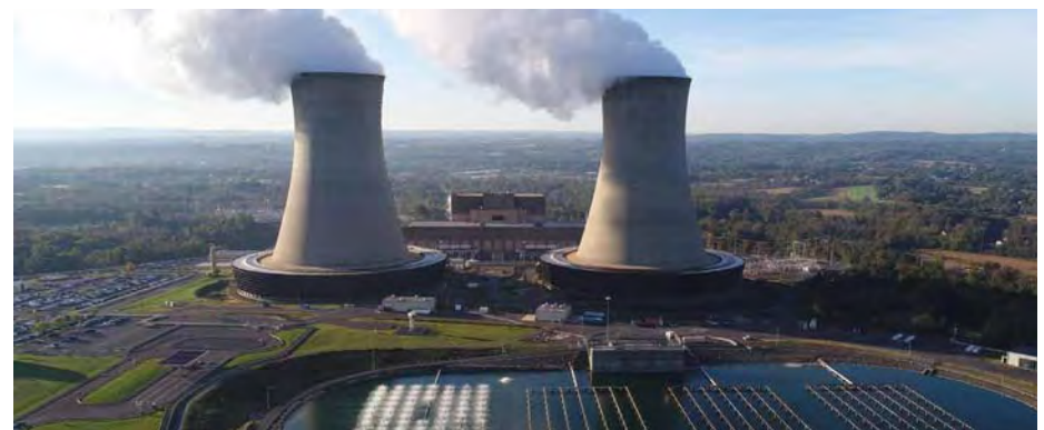
The Limerick Generation Station, located on the Schuylkill River in Pennsylvania, uses cooling towers to reduce the volume of cooling water needed.
